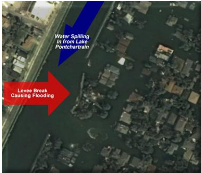
Figure 27: High-Resolution Imagery Using GeoFusion Showing a Major Levee Break and the Subsequent Flooding at a Location in New Orleans After Hurricane Katrina
