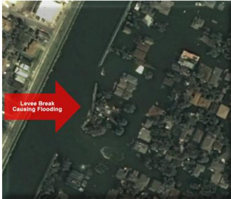
Figure 16: High-Resolution Imagery Using GeoFusion Showing a Major Levee Break and the Subsequent Flooding at a Location in New Orleans After Hurricane Katrina
